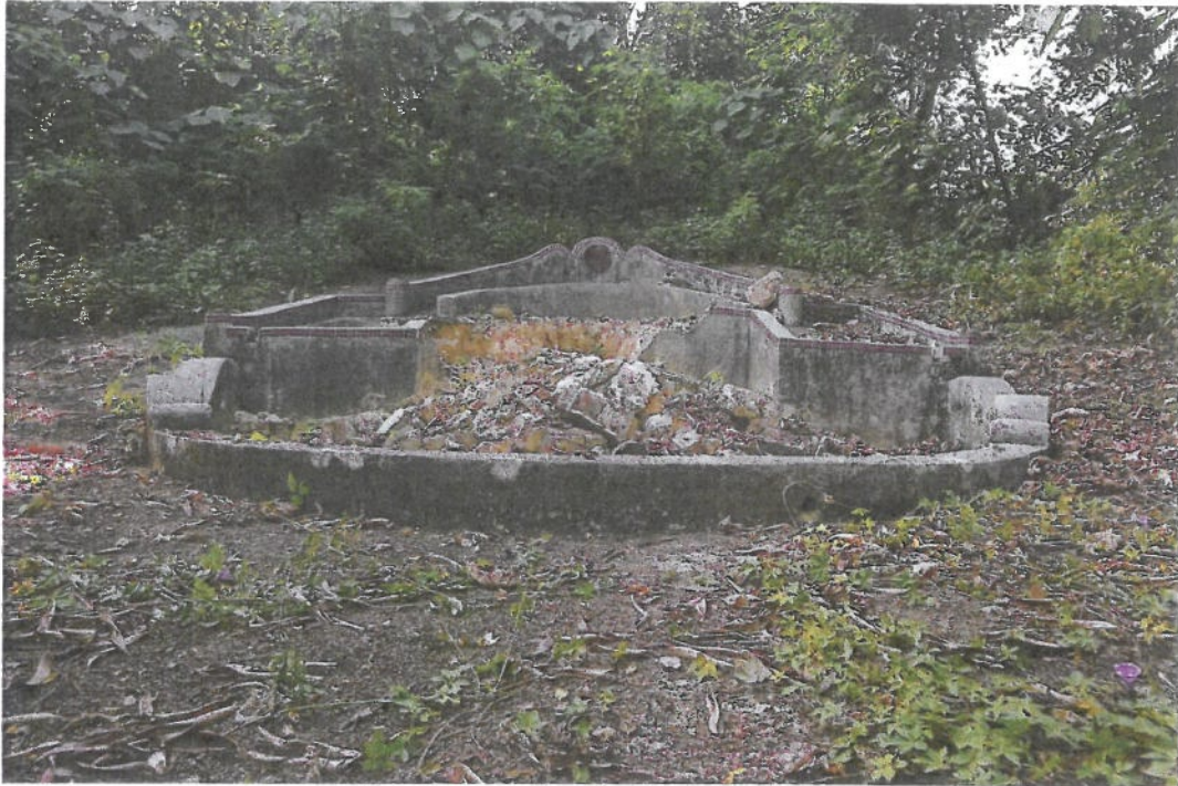
Photo 2: General View (Southeast to Northwest)
