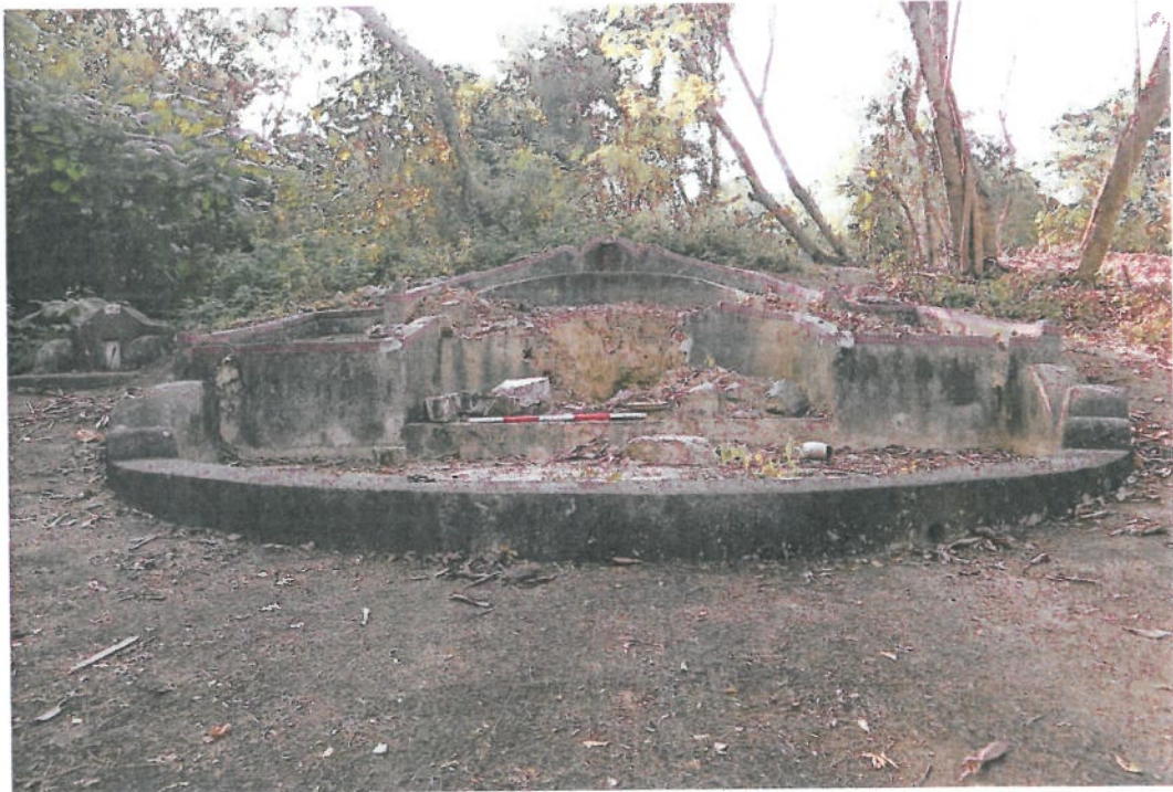
Photo 1: General View (East to West)
