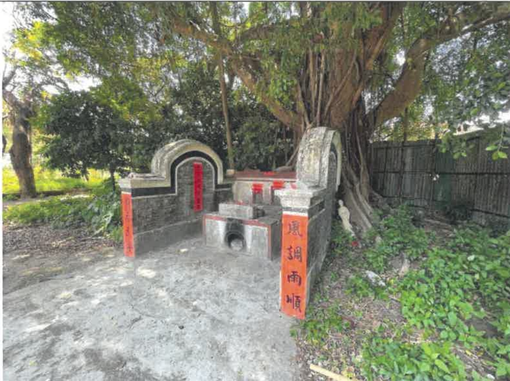
Photo : G202-2 (General View)
