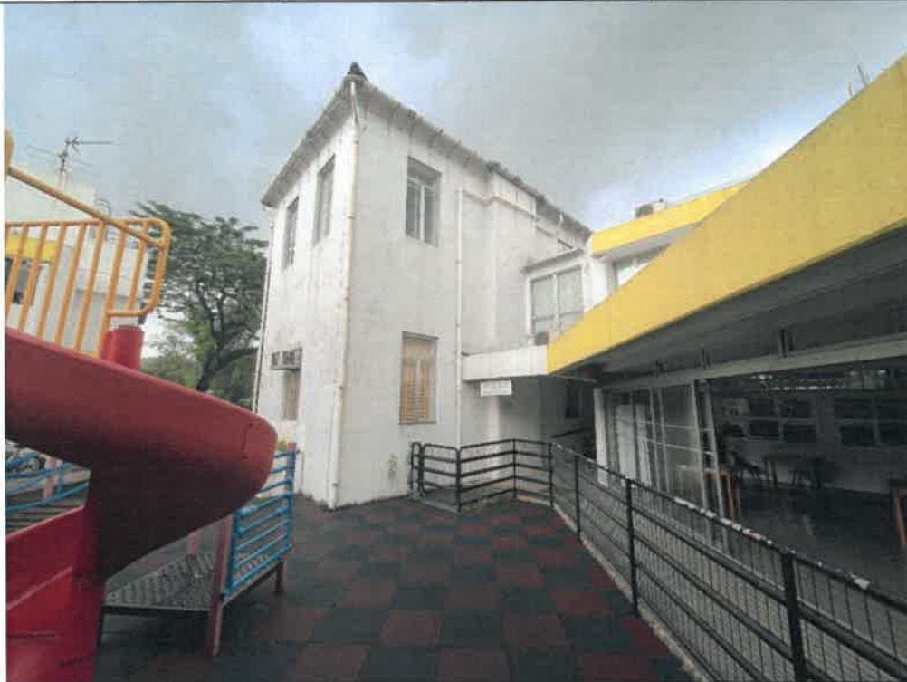
Photo: HKT03-03 Oblique View (North East to South West)
