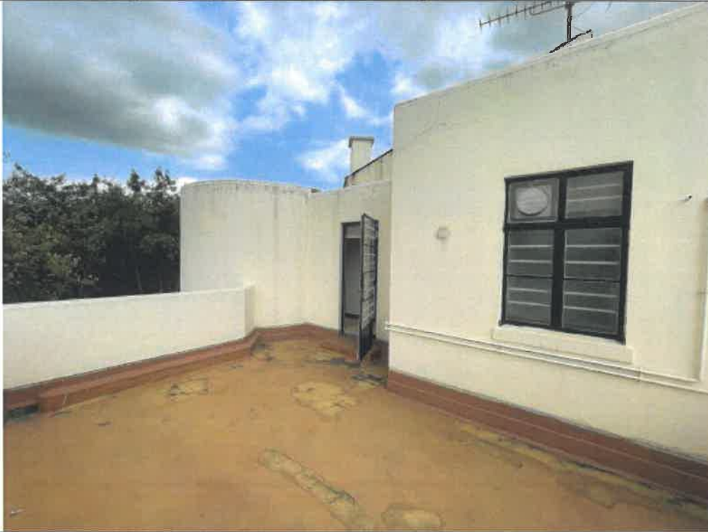
Photo: G303-33: 1/F Balcony
