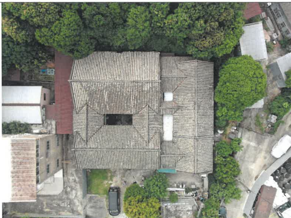
Photo G308-44: Top View (East to West)
