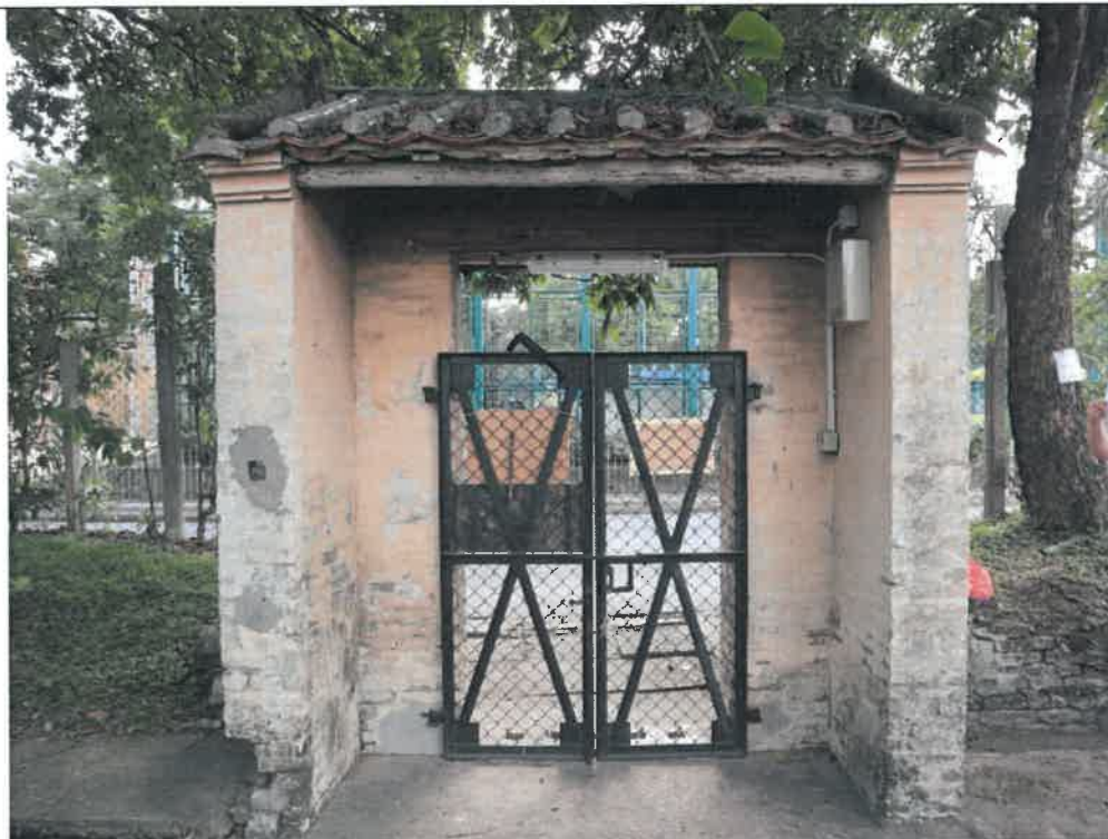
Photo 1- EG-2 Front View (East to West)
