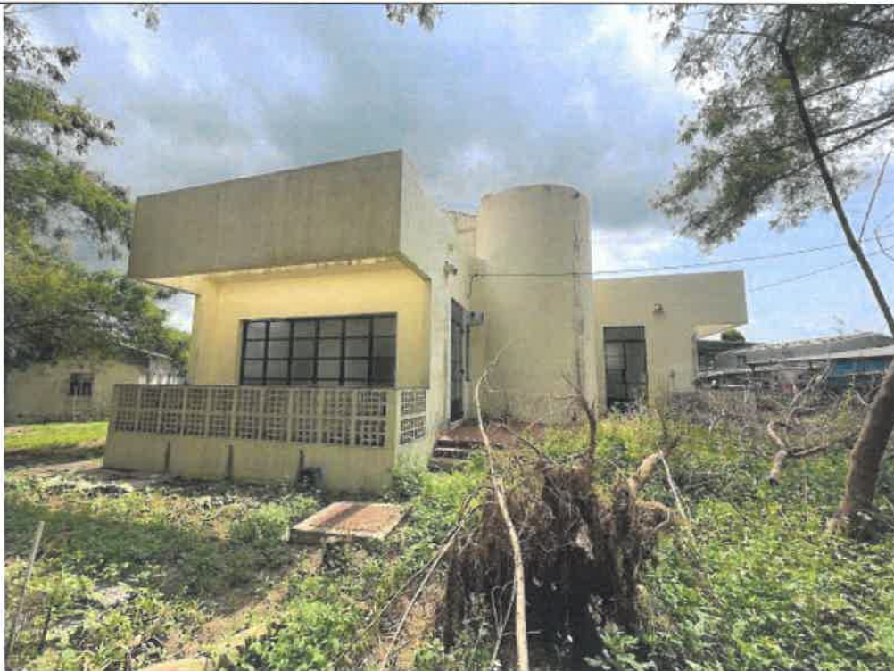
Photo: G303-6: Oblique View (North East to South West)
