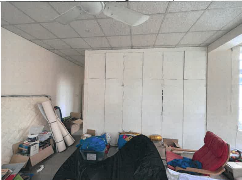
Photo: HKT03-35 Inside View
