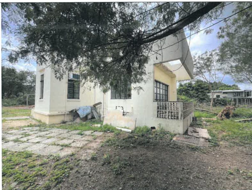
Photo: G303-4: Side View (East to West)
