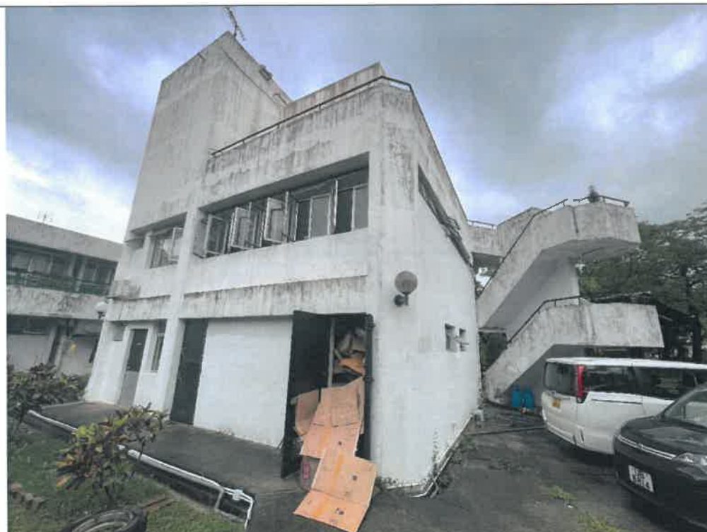
Photo: HKT03-12 Front View (North to South)
