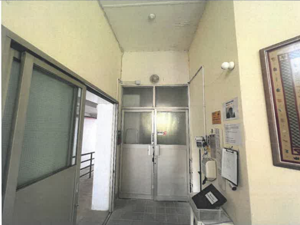
Photo: HKT03-25 Inside View
