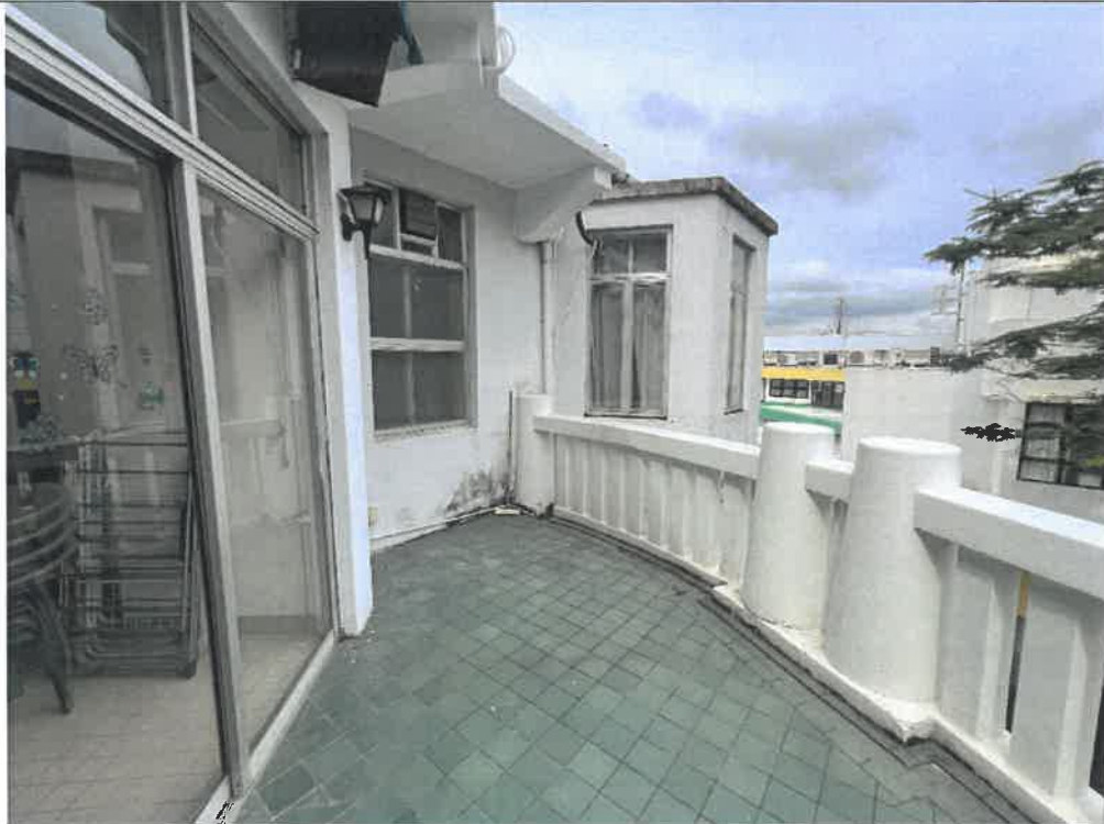
Photo: HKT03-50 Inside View
