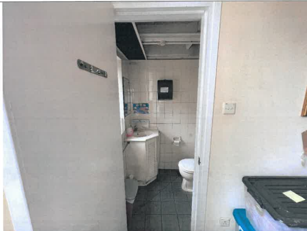
Photo: HKT03-16 Inside View
