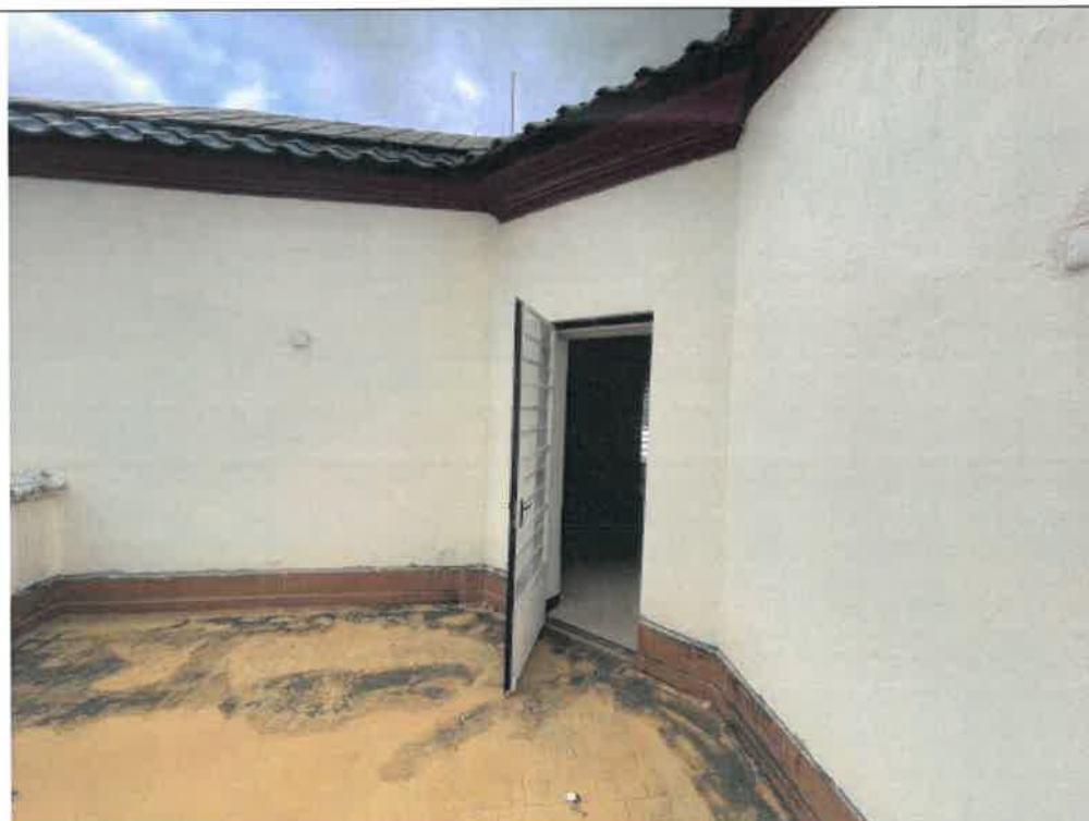
Photo: G303-32: 1/F Balcony
