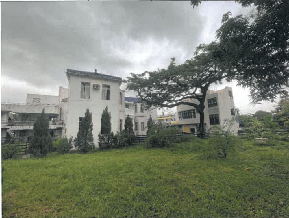
Photo: HKT03-07 Oblique View (South West to North East)
