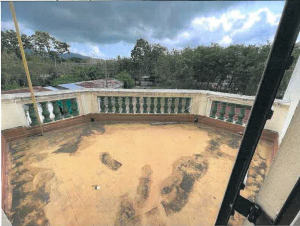
Photo: G303-27: 1/F Balcony
