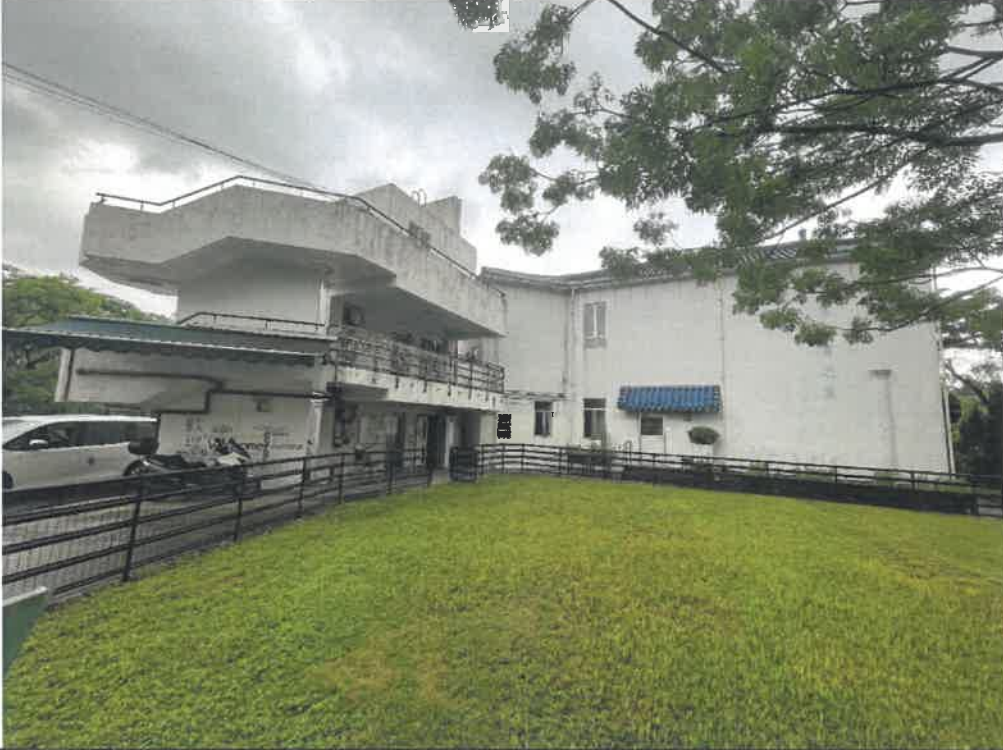
Photo: HKT03-09 Side View (West to East)
