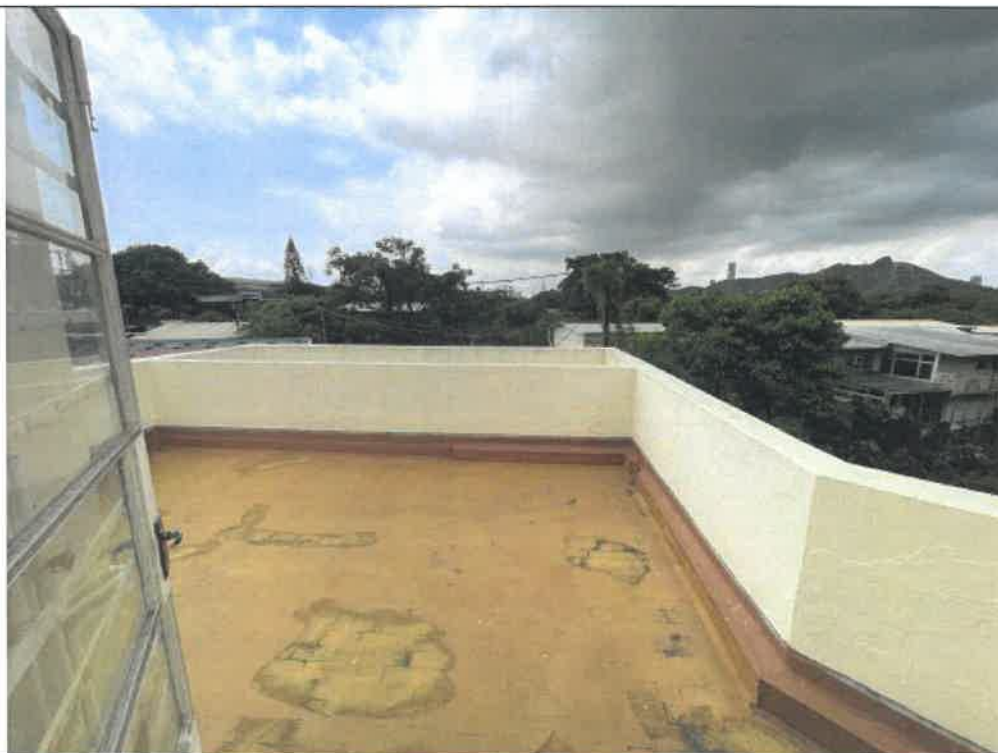
Photo: G303-30: 1/F Balcony
