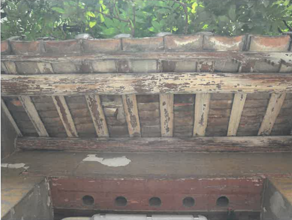
Photo 1- EG-7: Ridge of the entrance gate
