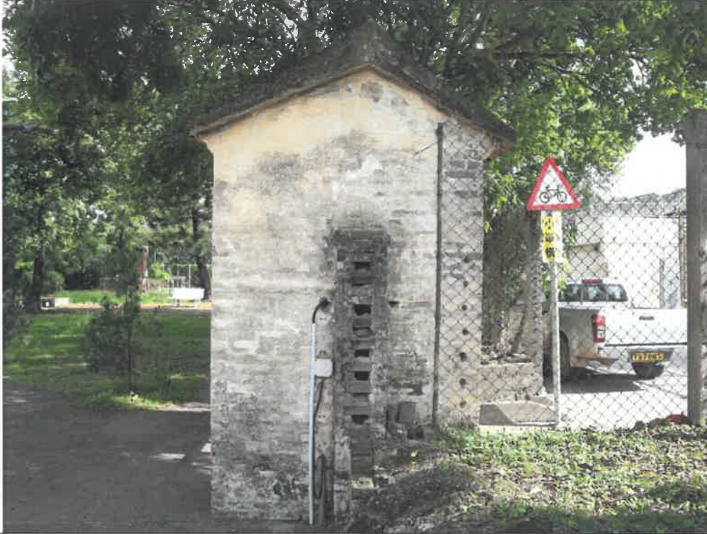
Photo 1- EG-3: Side View (North to South)
