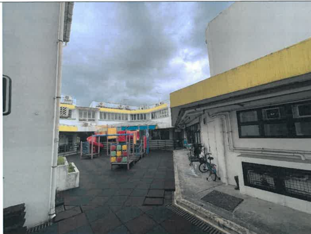
Photo: HKT03-04 Oblique View (South West to North East)
