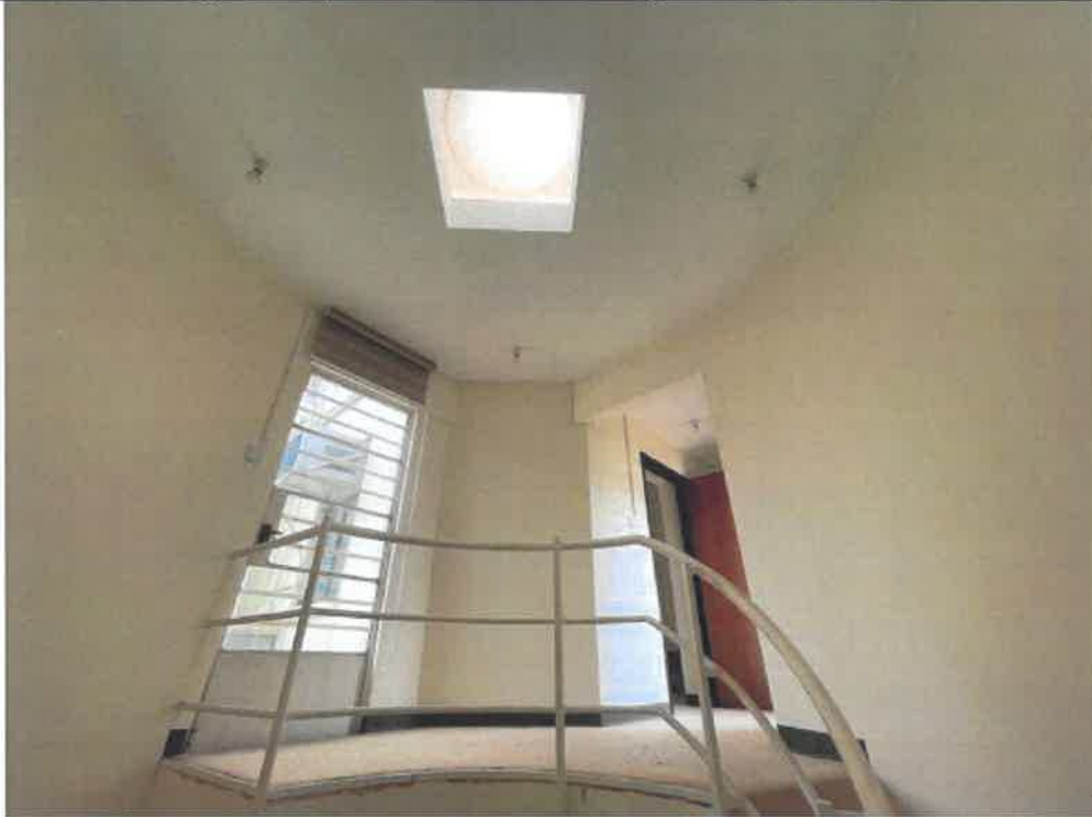
Photo: G303-21: 1/F Staircase
