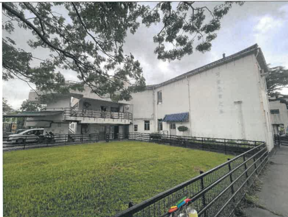
Photo: HKT03-08 Oblique View (South West to North East)
