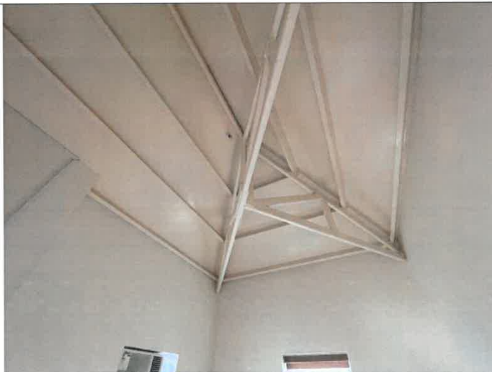
Photo: G303-24: 1/F Bedroom Ceiling
