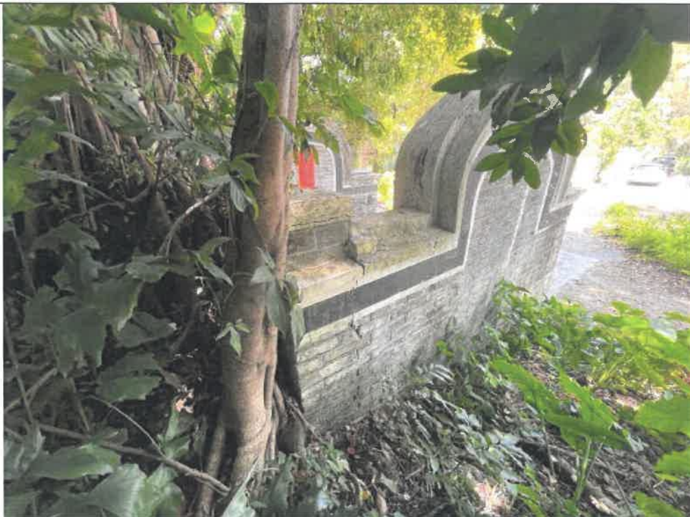
Photo : G202-6 (General View)
