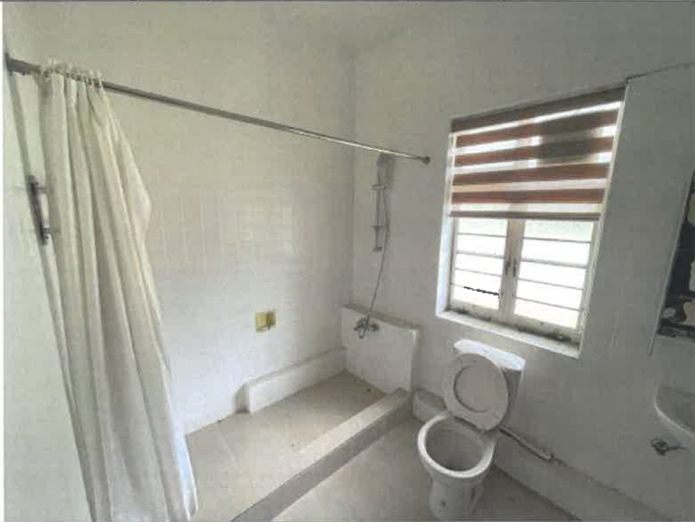
Photo: G303-25: 1/F Toilet
