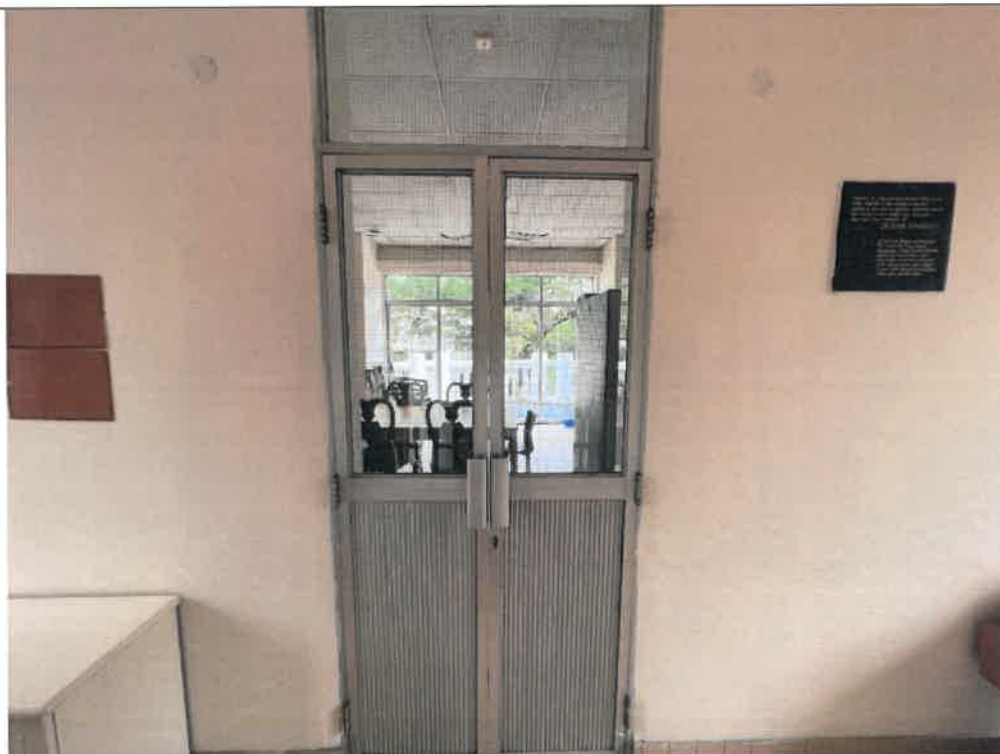
Photo: HKT03-44 Inside View
