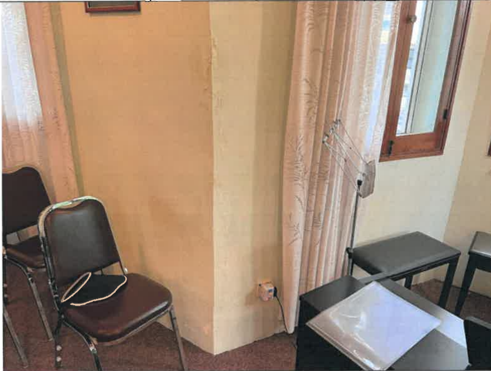
Photo: HKT03-23 Peel off paint with mositure
