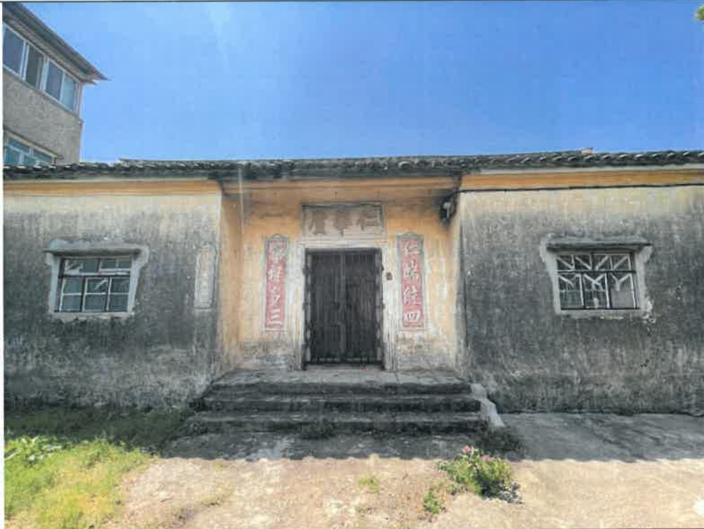
Photo G308-1: Front View (East to West)
