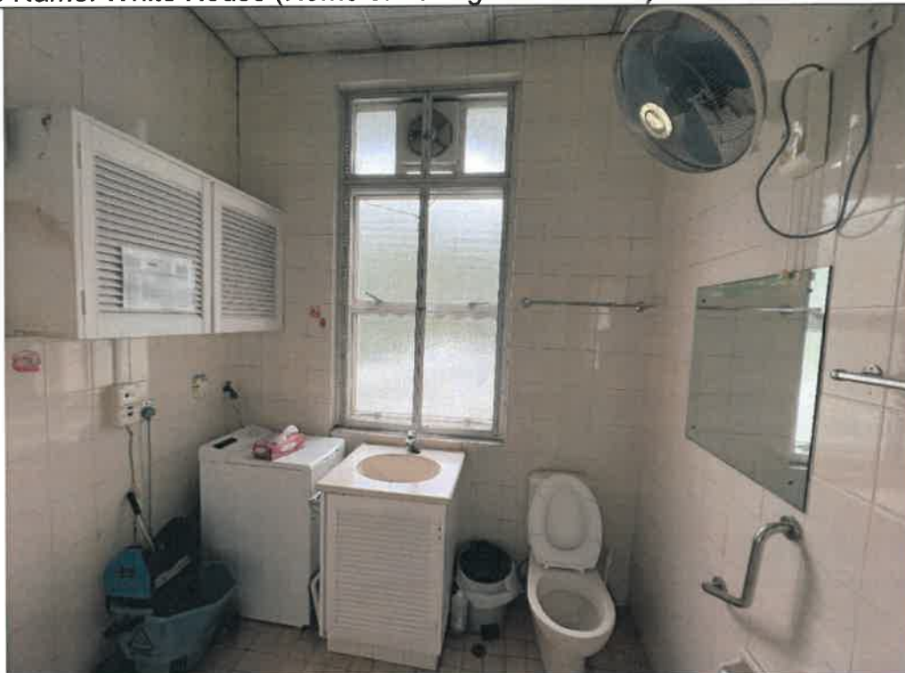
Photo: HKT03-43 Inside View
