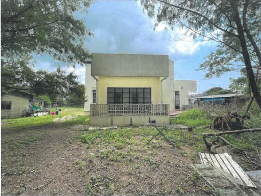
Photo: G303-5: Oblique View (North East to South West)
