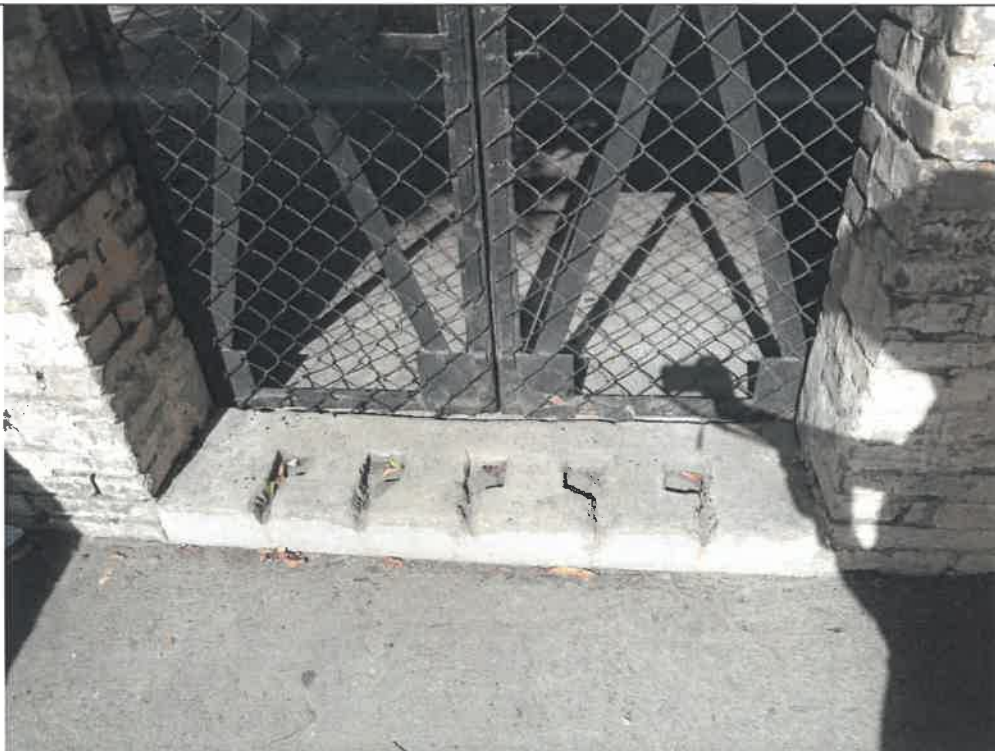
Photo 1- EG-8 Stone base of the entrance gate
