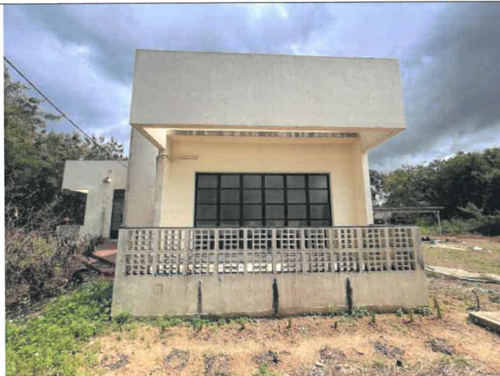
Photo: G303-8: Oblique View (North West to South East)
