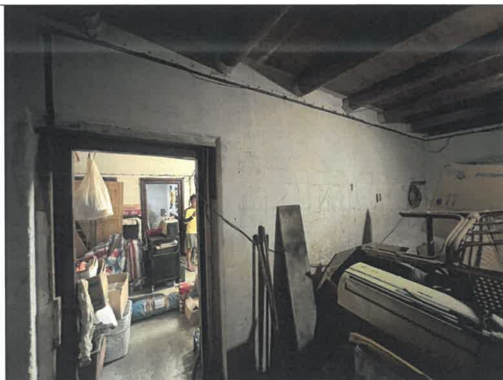
Photo G308-20: Inside View
