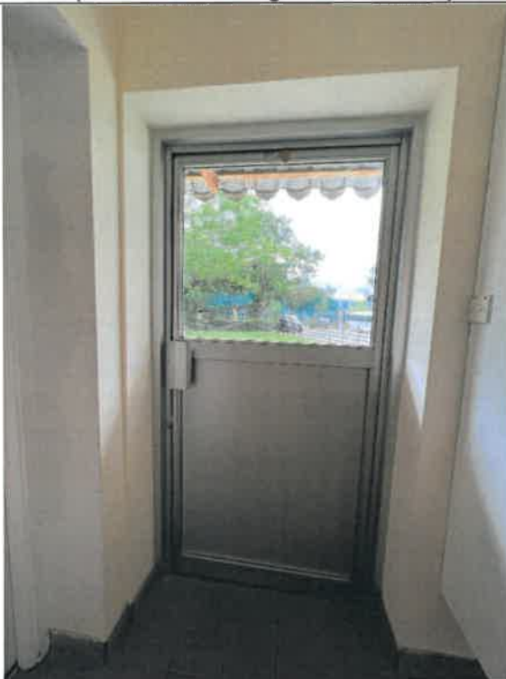
Photo: HKT03-19 Inside View
