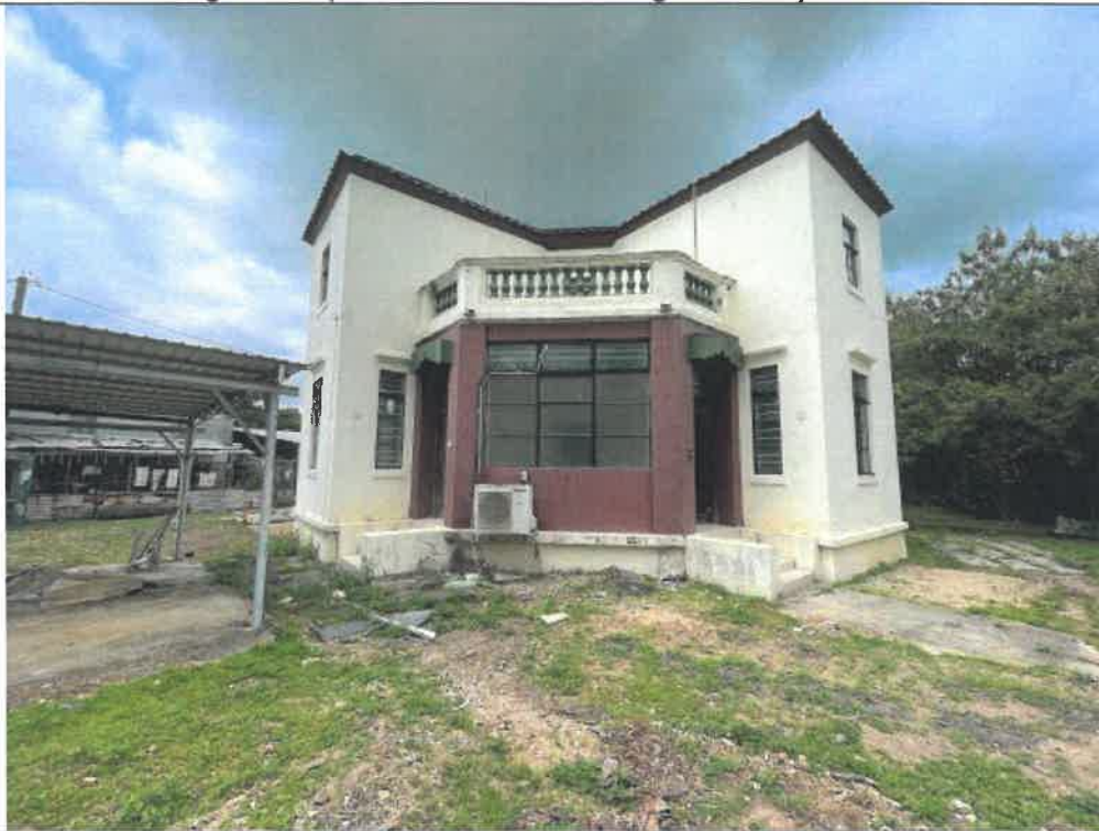
Photo: G303-1: Front View (South to North)
