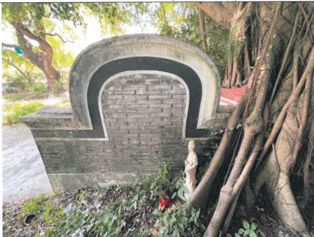
Photo : G202-3 (General View)
