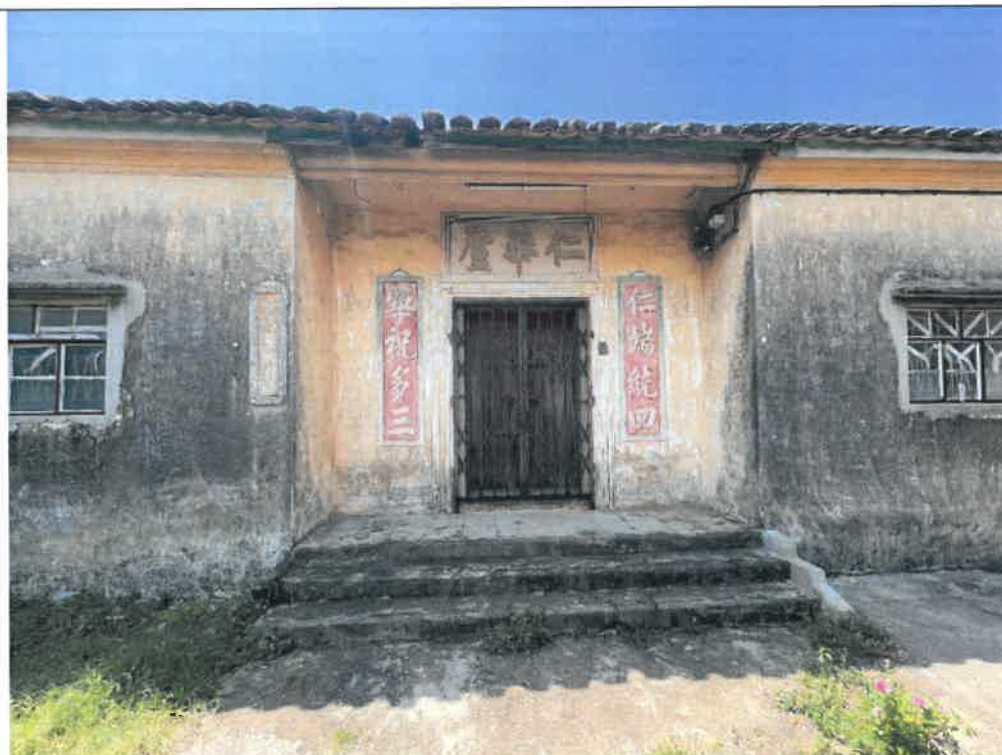
Photo G308-2: Front View (East to West)
