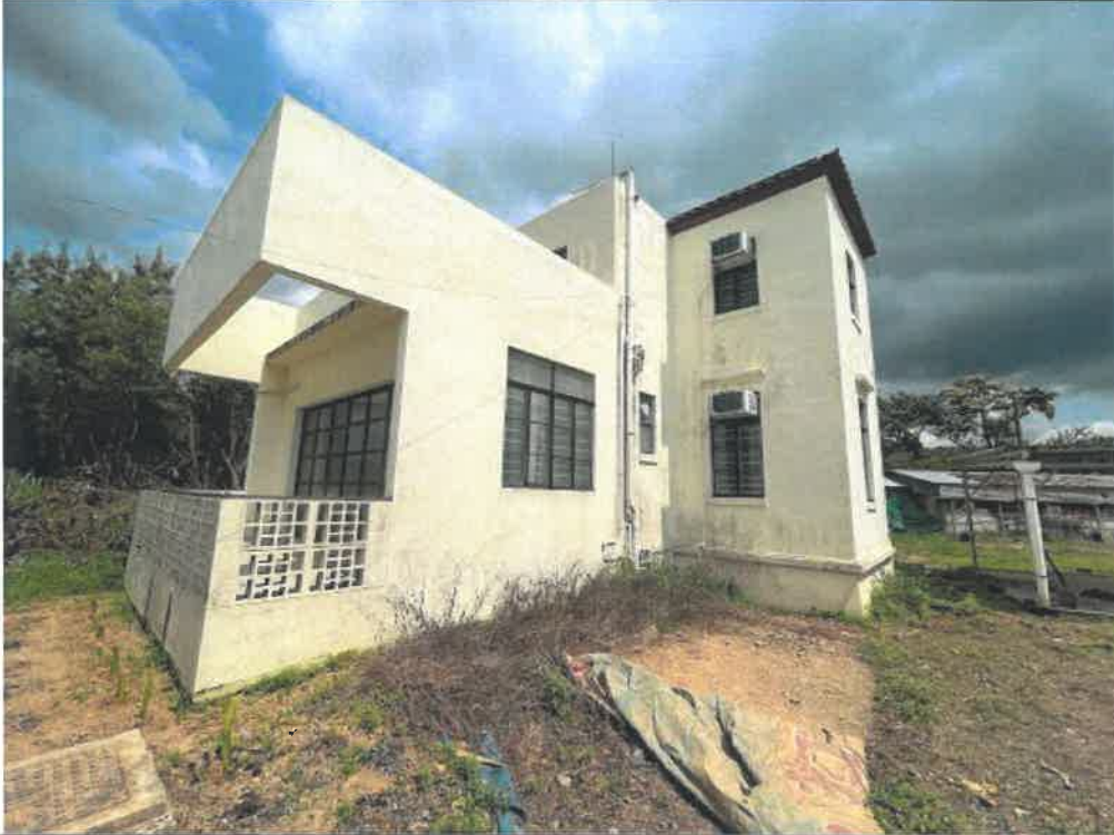
Photo: G303-9: Side View (West to East)
