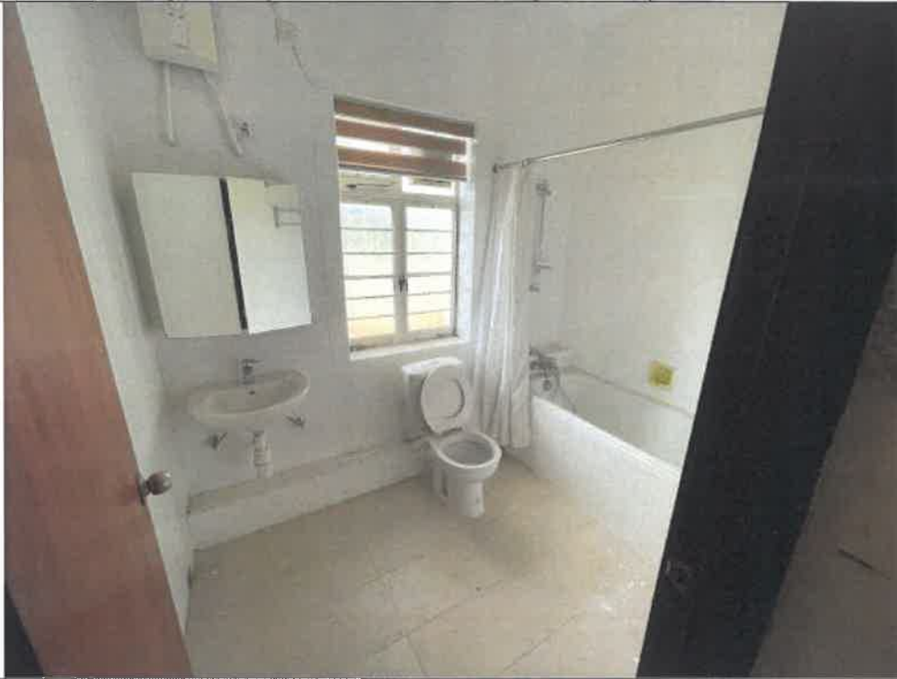
Photo: G303-29: 1/F Toilet
