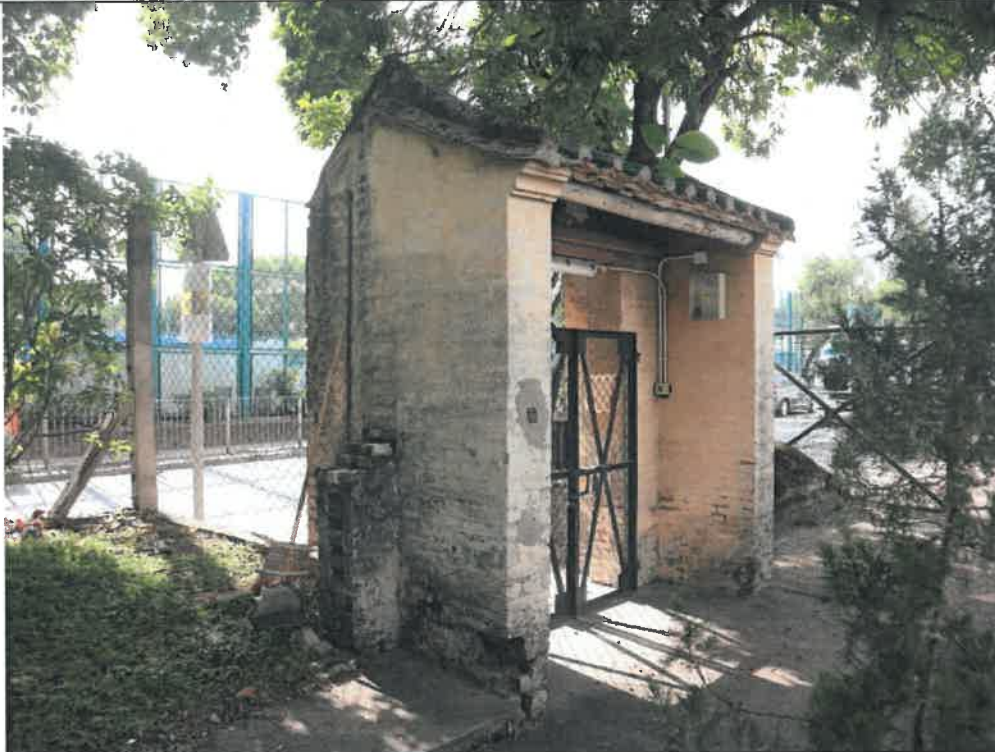
Photo 1- EG-5: Oblique View (South East to North West)
