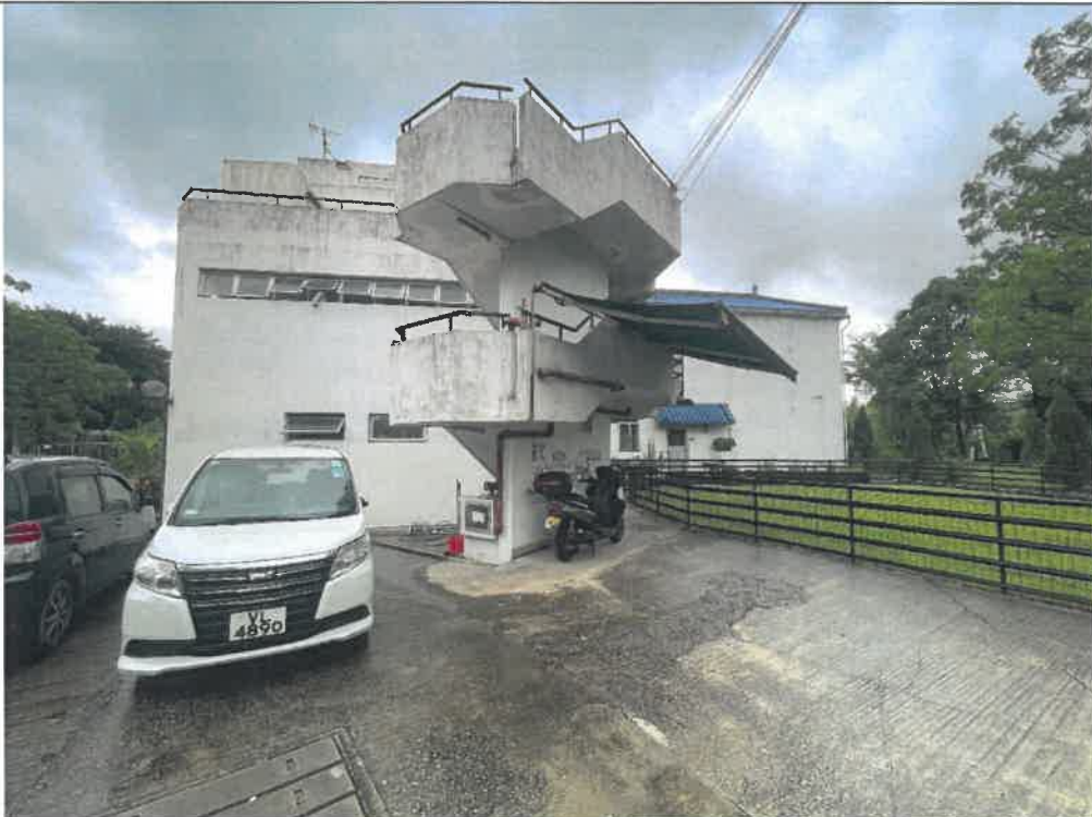
Photo: HKT03-10 Side View (West to East)
