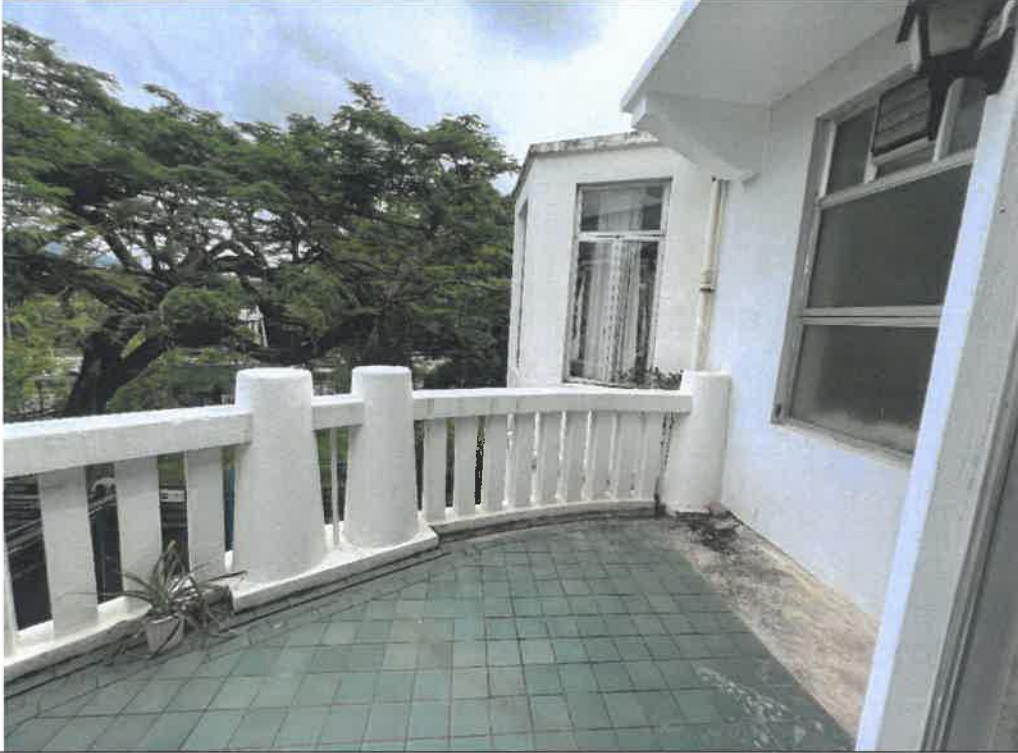
Photo: HKT03-49 Inside View
