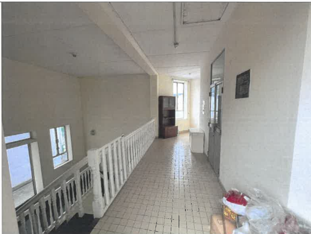
Photo: HKT03-38 Inside View
