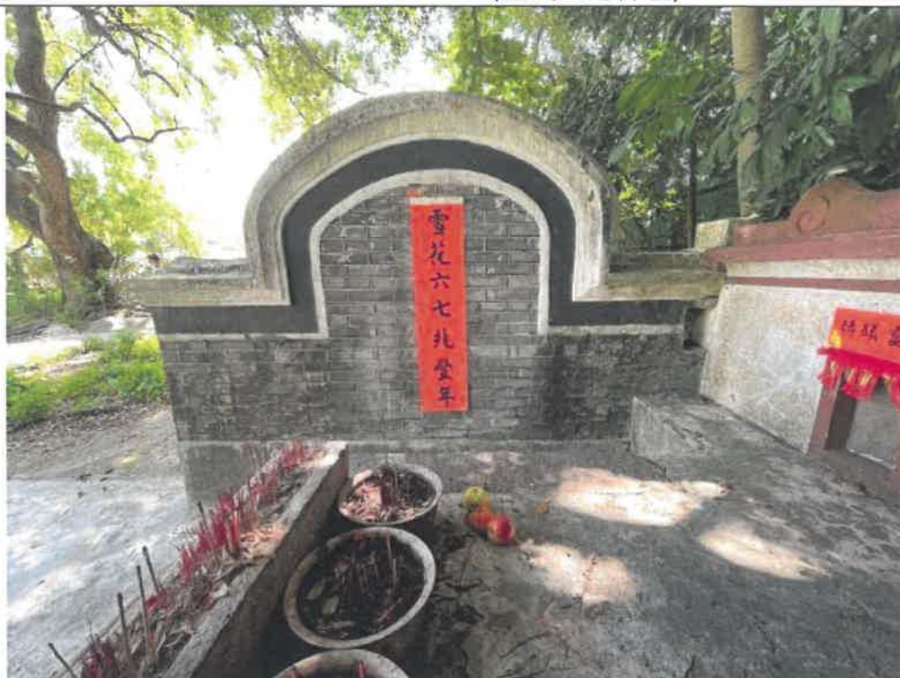
Photo : G202-9 (General View)
