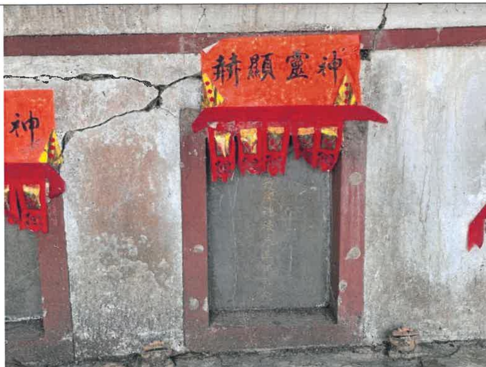
Photo : G202-8 (General View)
