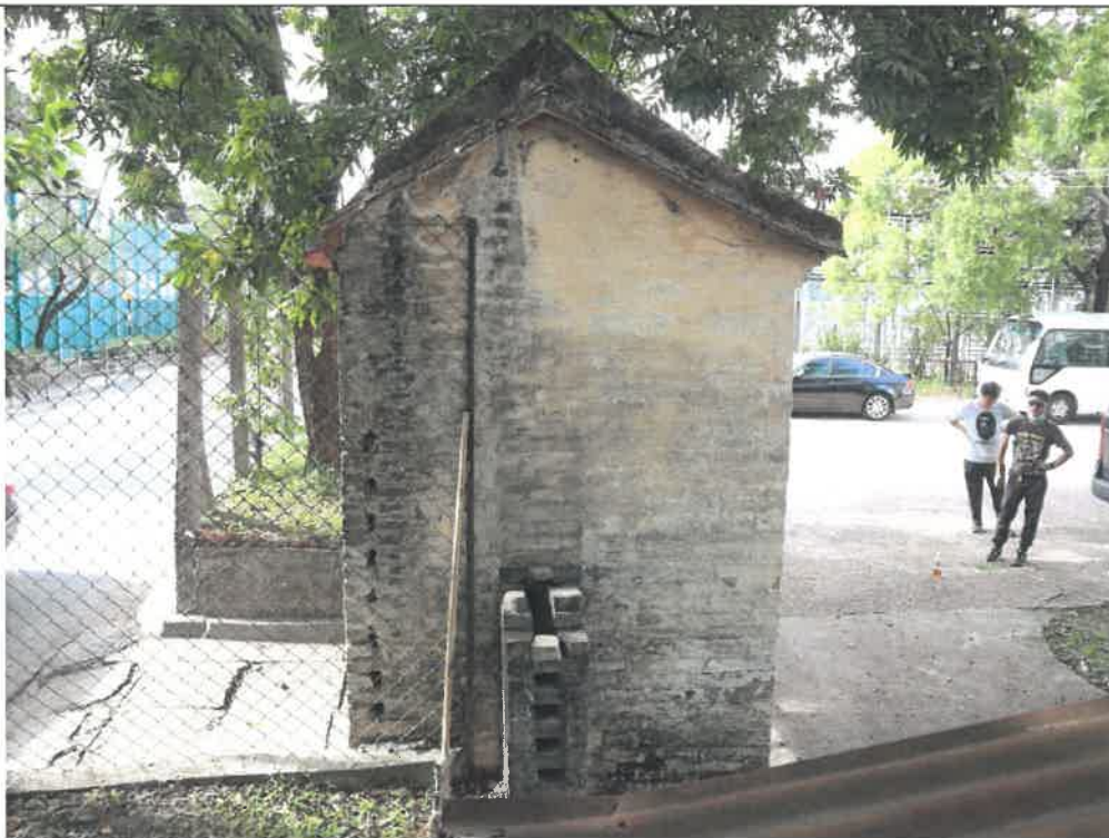
Photo 1- EG-4 Side View (South to North)
