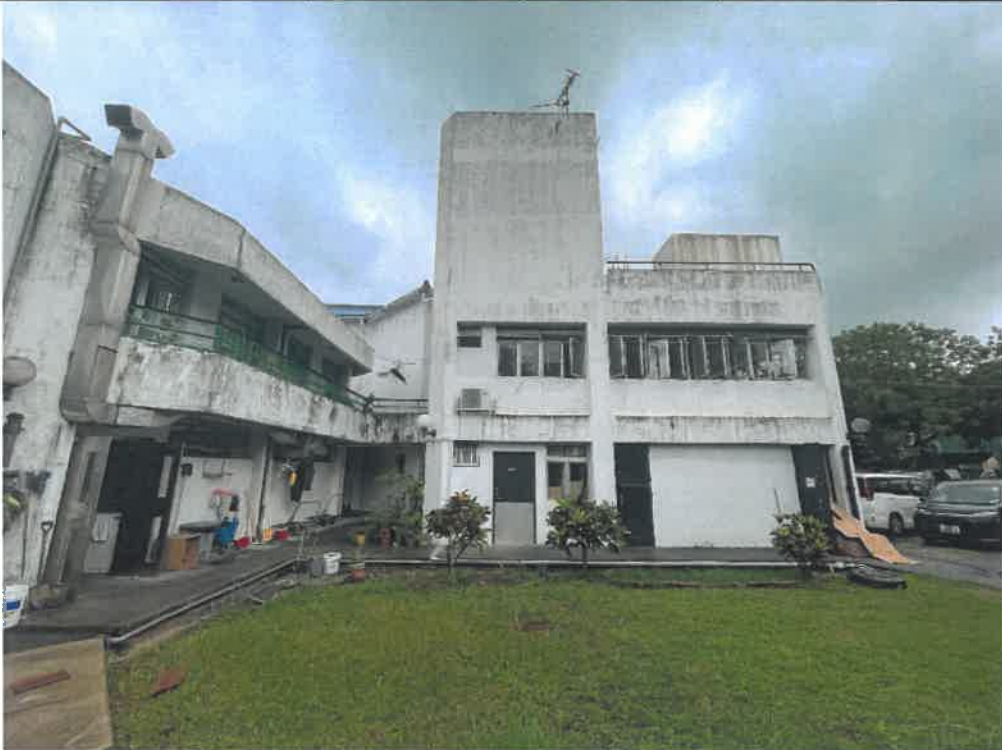
Photo: HKT03-13 Oblique View (North East to South West)
