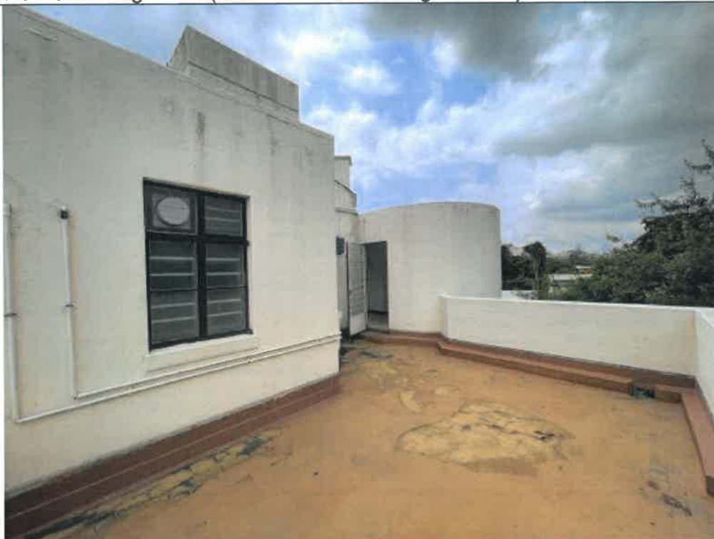
Photo: G303-31: 1/F Balcony
