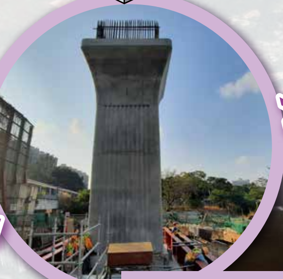
橋墩施工 Bridge pier construction
